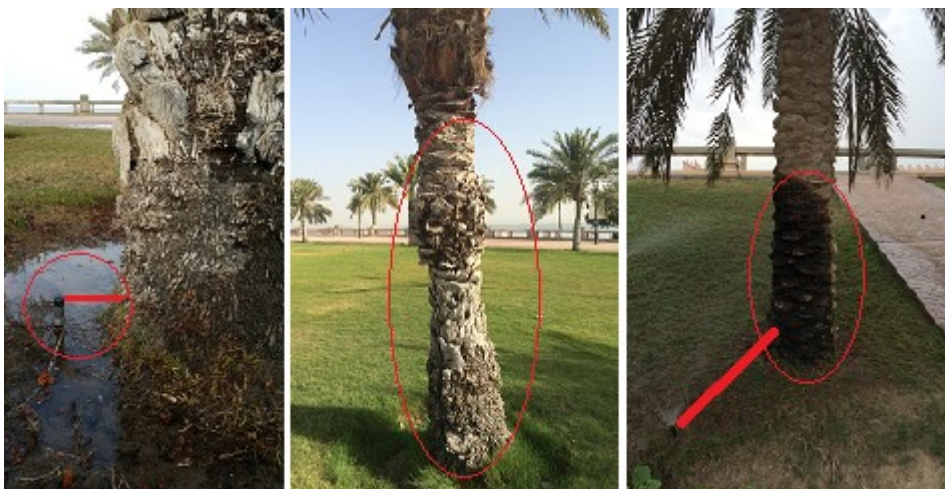
Figure 6: The placement of irrigation dischargers (bubblers 10-30 cm and closer to the palm tree and sprayers are continuously spraying the trunk) cause serious effects.
