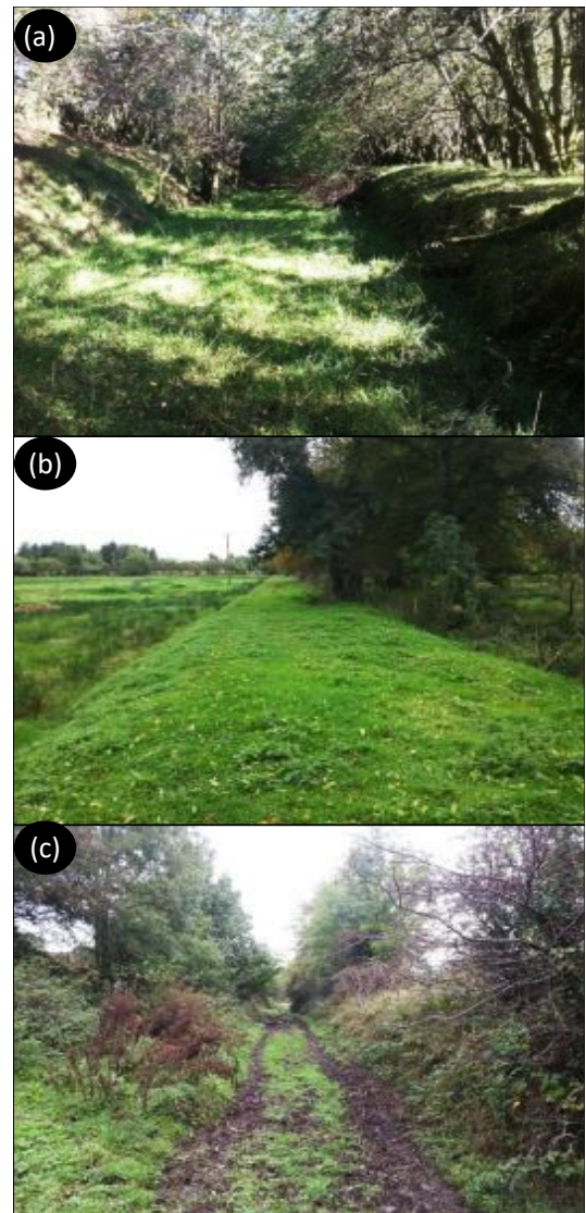
Figure 5: (a) Railway bench- cut section with overgrown hedgerows bounding both sides and semi-natural grassland blanketing the ballast; (b) Grazed railway embankment with mature and overgrown hedgerow bounding one side; (c) Railway cut section with remnant gappy hedgerows and poaching of ballast surface by livestock.
