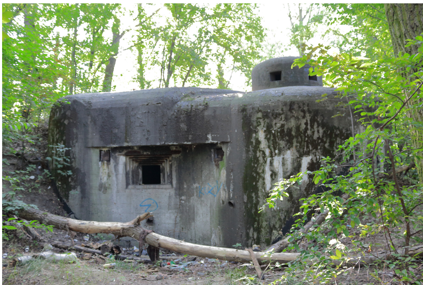
Figure 5. Heavy battle bunker of the Warring Area ‘Śląsk’. (Photo: Rostański K.M.).
